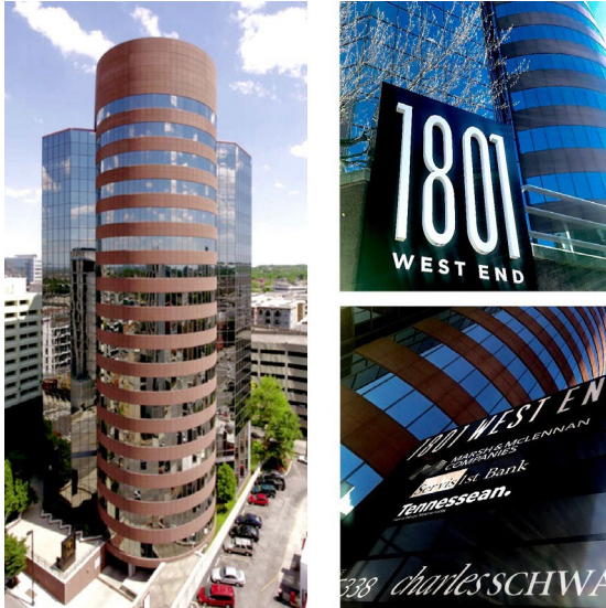
1801 West End Ave. Building view from West End
